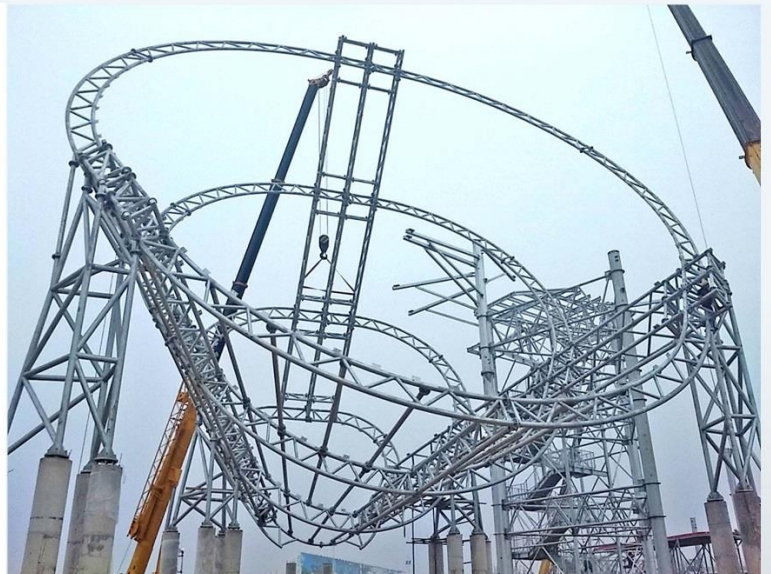
NSS Abyss structure installed on site
